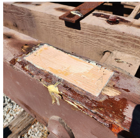
Right: AFTER - The top of the sill after the splice and epoxy. The last step was to sand it smooth.
