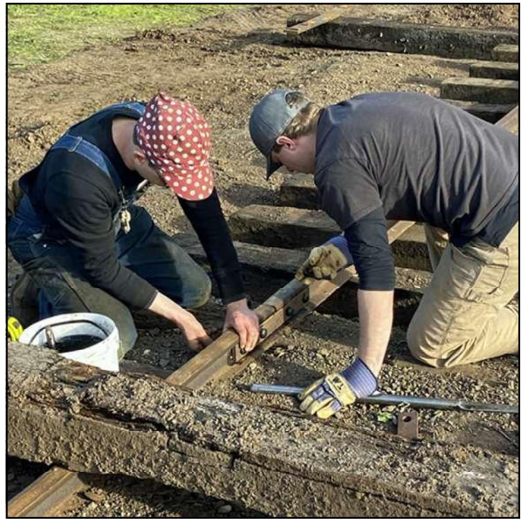
Bobby Goldie (right) and David Waterman (left) work on the new spring switch at Shirley's Siding (2/19/23). Photo by John Goldie
