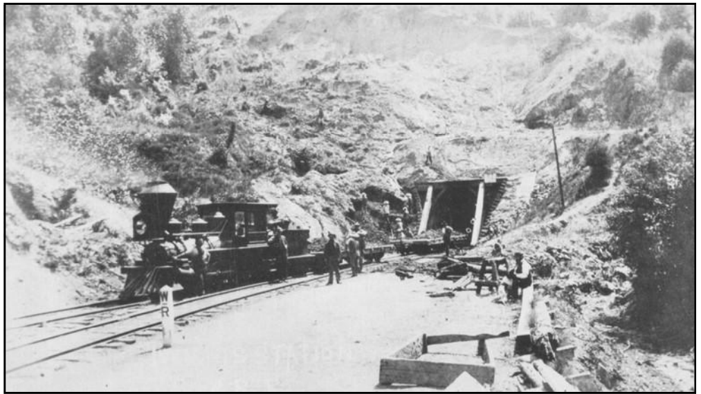
Wright's Portal, Tunnel 2, December 1893.
