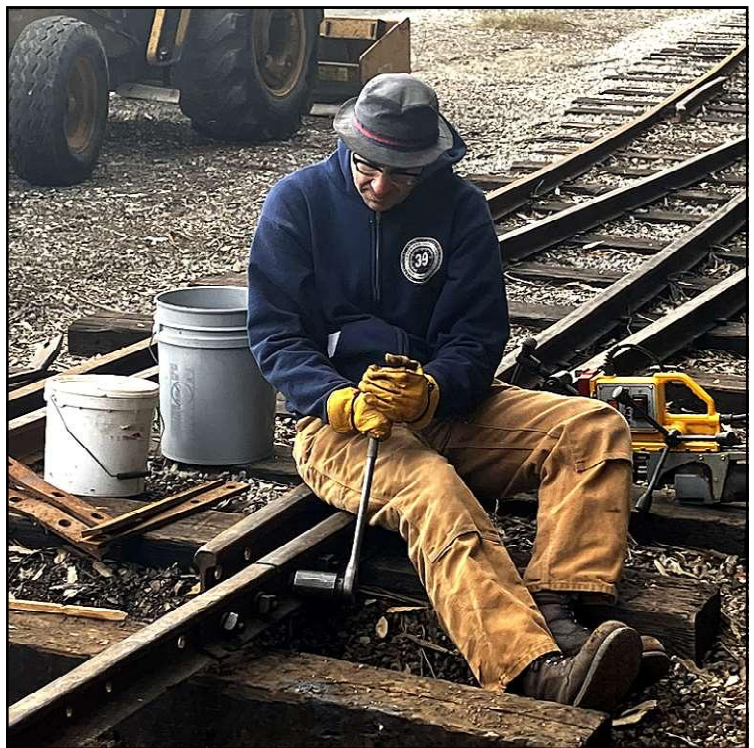
Spring Switch Deer Park East-Damian Stellabott tightens the track bolts (1/29/23). Photo by John Goldie
