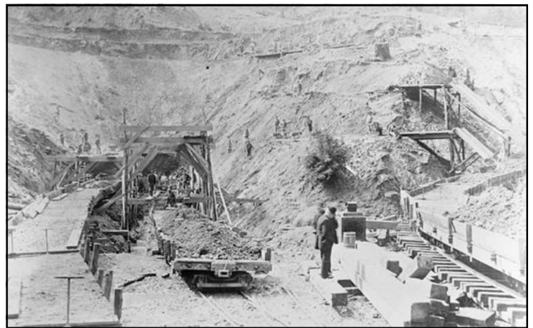
Wright's Tunnel Portal, March 1893. Bruce MacGregor Collection
