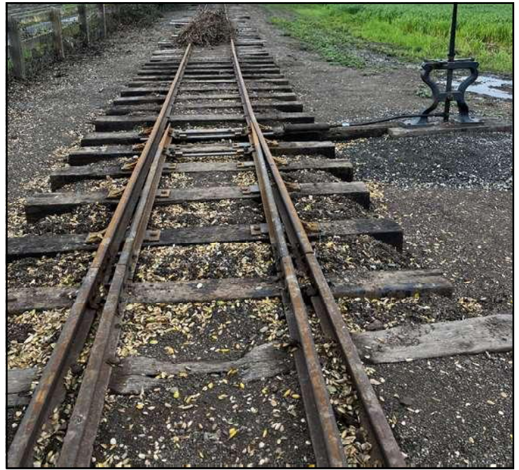
Spring switch at Shirley's Siding is almost complete.
