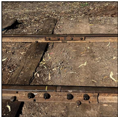
Rail joint with key rail (2/12/23).
