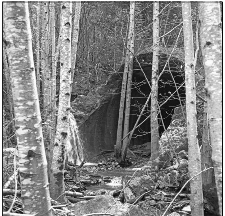
Wright's Portal, Tunnel No. 2, 1967.
