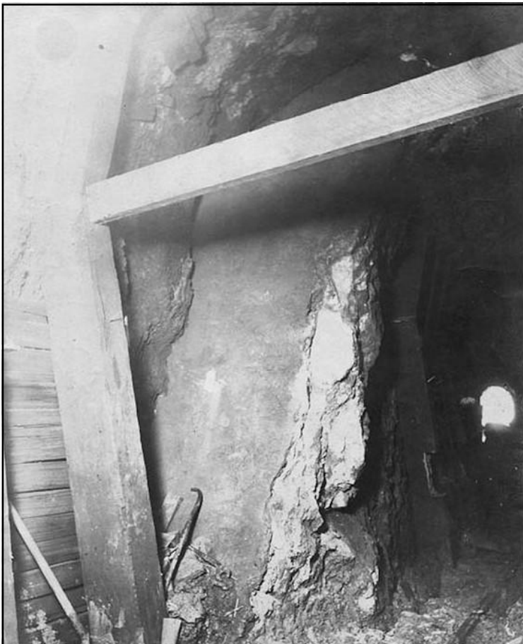
San Andreas Fault offset in tunnel No. 2, 1906. Wright's tunnel portal in the distance. John Hall Collection
