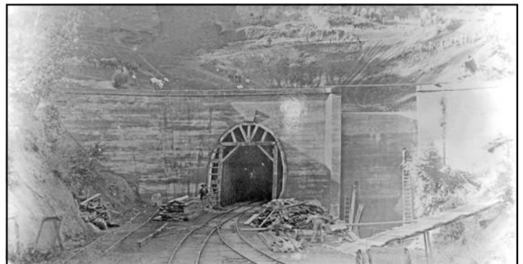
Wright's Tunnel Portal with falsework, Fall 1893.
