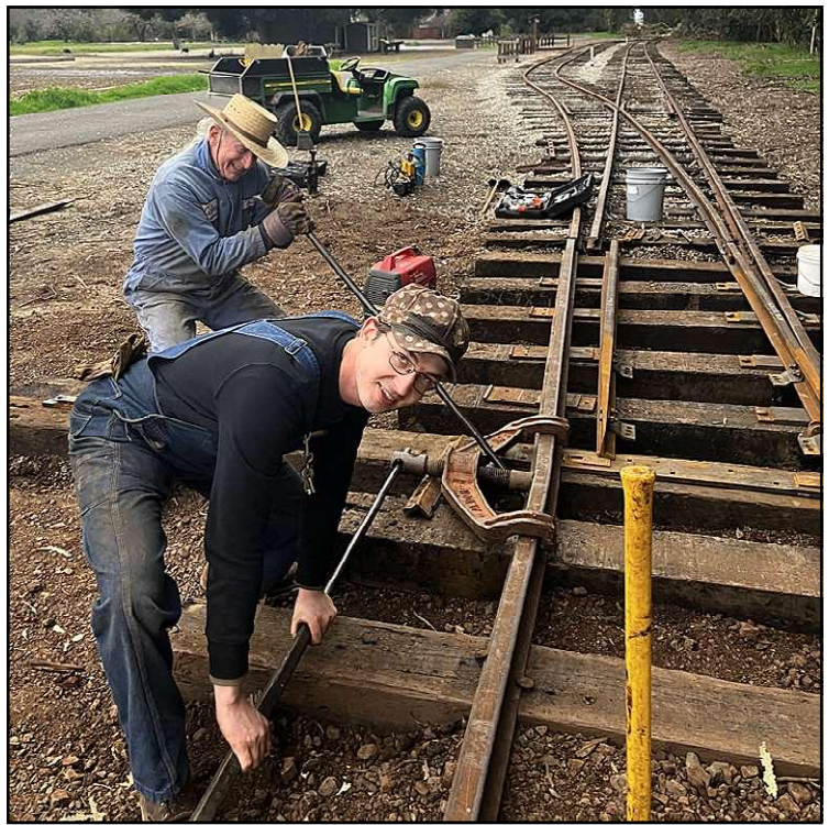
Spring Switch Deer Park East-David Waterman (front) and Bruce Sorel put the bend into the curved stock rail just ahead of the point tip (1/29/23). Photo by John Goldie
