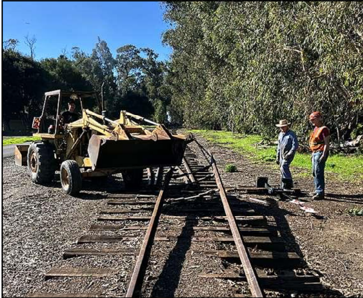
Spring switch at Deer Park east. David Waterman lifts out the swing rails as Bruce Sorel and Steve Rusconi direct (01/22/23).
