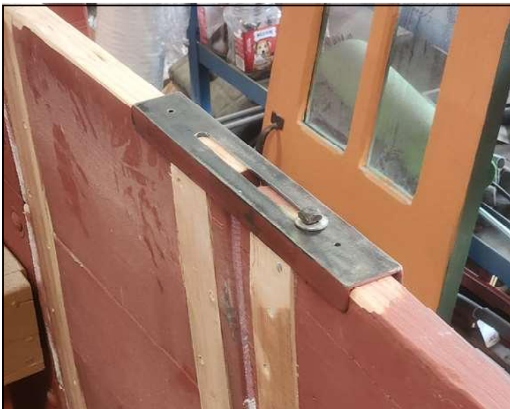
Here are the doors with the hardware installed.
