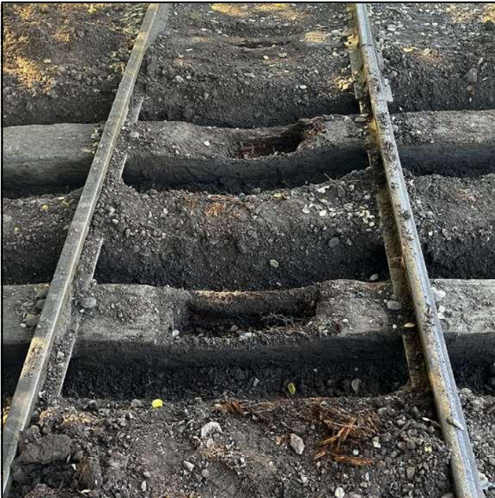
Years of horse power have worn out the middle of many ties, thus it is time for a change out.
