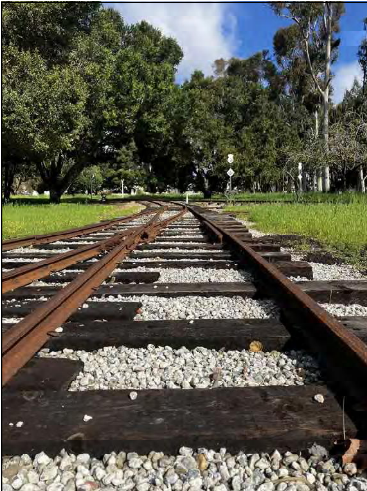
An active project for April is to connect up this harp stand - it will lead to additional yard tracks.
