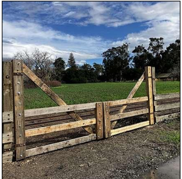
New gates replaced the old, rotted gates. This now gives us direct access to the track.
