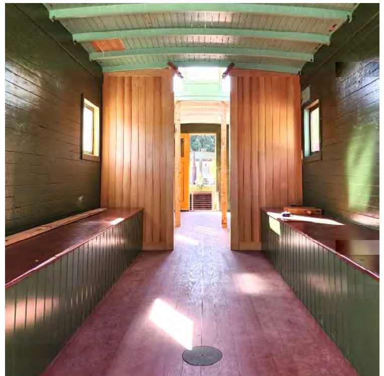
Benches complete and partitions going in.
