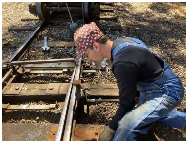
David Waterman working on the Deer Park west spring switch. Photo by John Goldie
