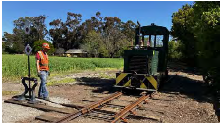
Testing the switch - no more joint kinks
