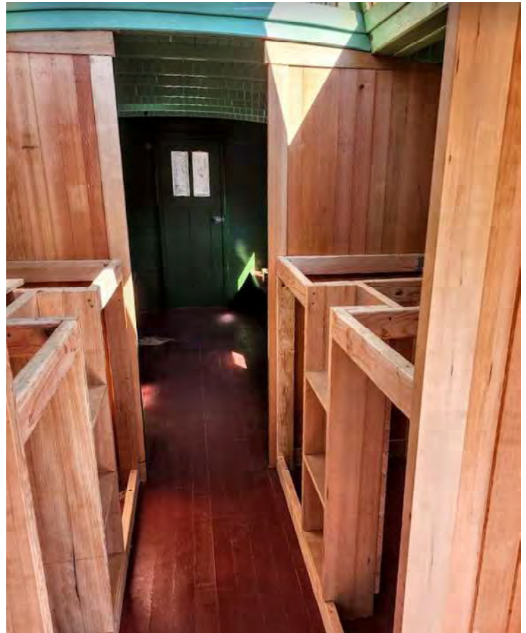
Cabinets and stairs to cupola are framed and partially sheathed.
