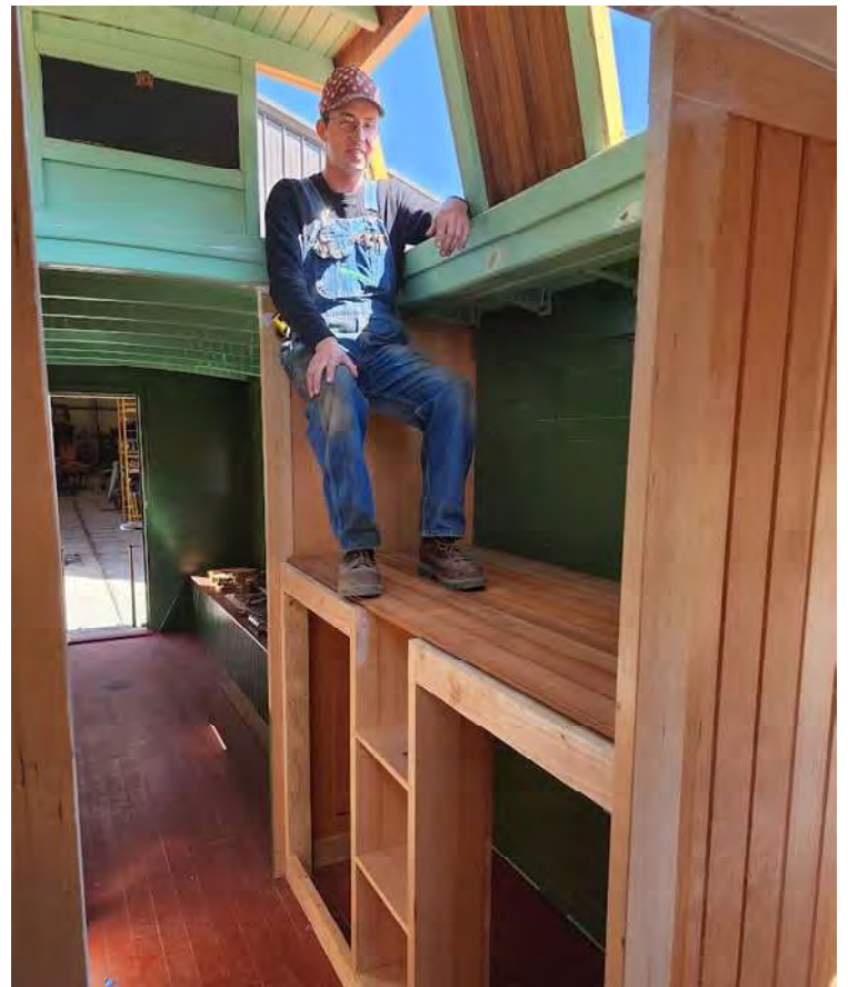
David in 'air seat' testing for how high to make cupola seats.
