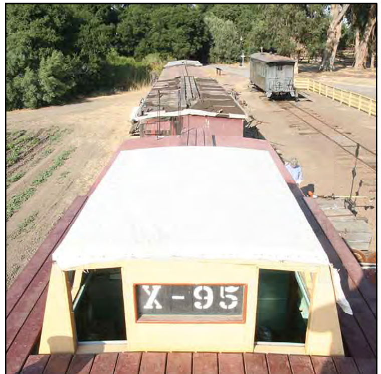
New canvas roof being fitted for NWP caboose 6101's cupola.
