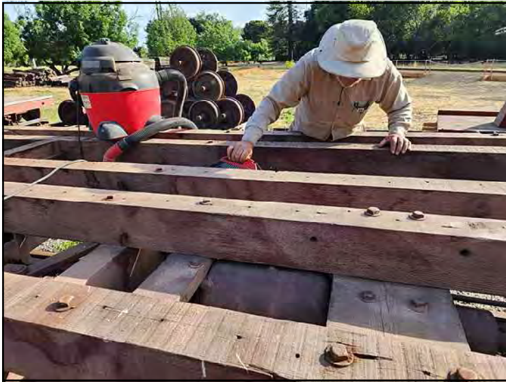
John Stutz inspects the wood on NS 1725.
