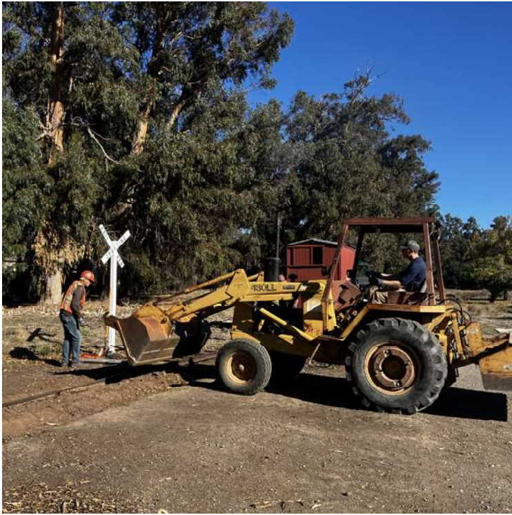
Steve Rusconi spots David Waterman in the tractor working on the rebuilt crossing. Next step is to install the new planks.
