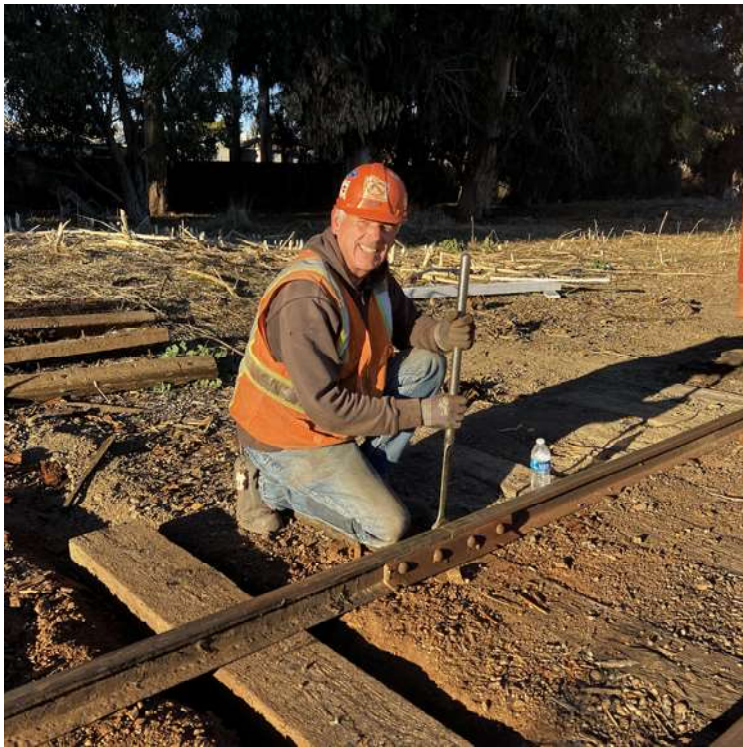
Steve Rusconi bolting a joint bar after the crew replaced the tie at this location.
